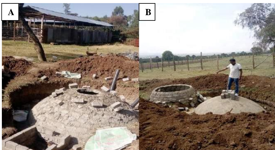
FIG. 2.A.B. A 10 m 3 fixed dome bio-digester abebech gobena research center (AGRC), Birbirsa
