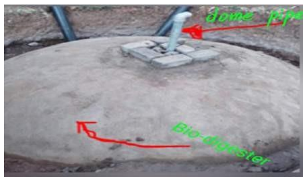
FIG. 3. A 10 m 3 fixed dome bio-digester at AGRC , birbirsa (after construction, 2022)
