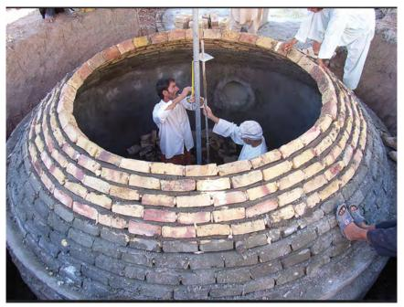
FIG. 69. A dome under construction.
