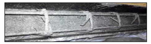
Fig. 2: Casting of SIFCON beam
