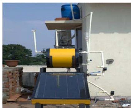
Fig. 1: 25 LPD collector with primary riser tube and secondary storage tank
