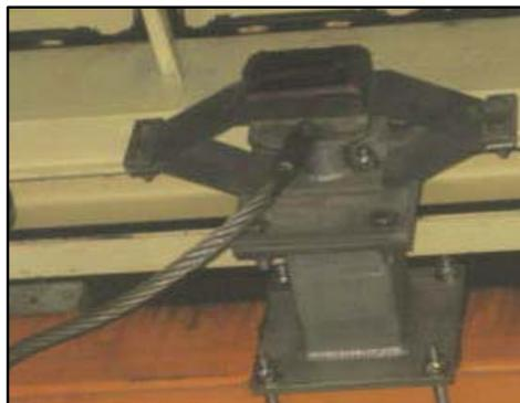
**Fig. 9: Cathode connection**
