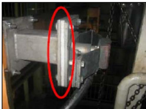
**Fig. 10: Insulator in bus bar**
