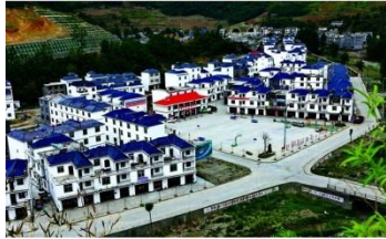
Figure 4: (Upper one) Zaoshu resettlement community, baihe
