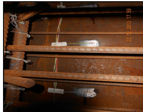
Fig. 5: Field photo: Strain gauges in the girder at site
