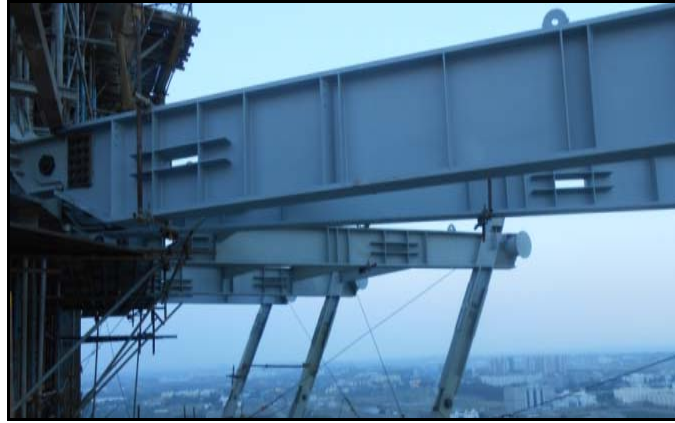
Fig. 3: Field photo: Anchorage system at 102 m
