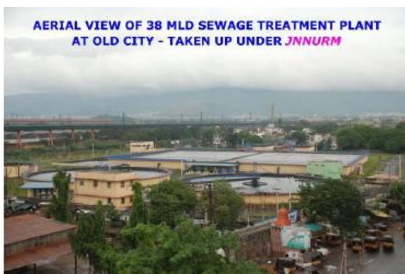
Figure 1 : 38 MLD sewage treatment plant at old city
