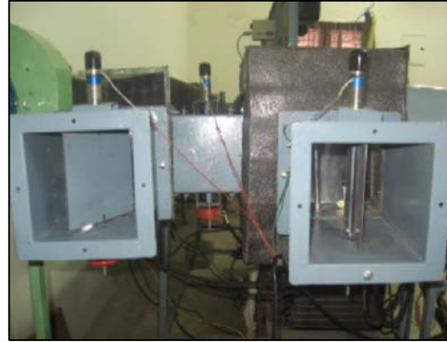
Fig. 7: View of supply and return duct system
