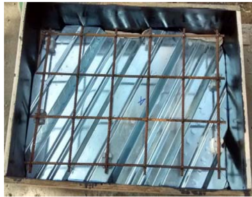
Fig. 3: Photograph of 30° profiled steel deck slab
