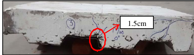
Fig. 10: Slip behaviour for slab 0°
