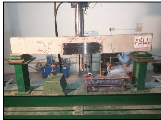
Fig. 7: Cracking pattern of ASW-F specimen
