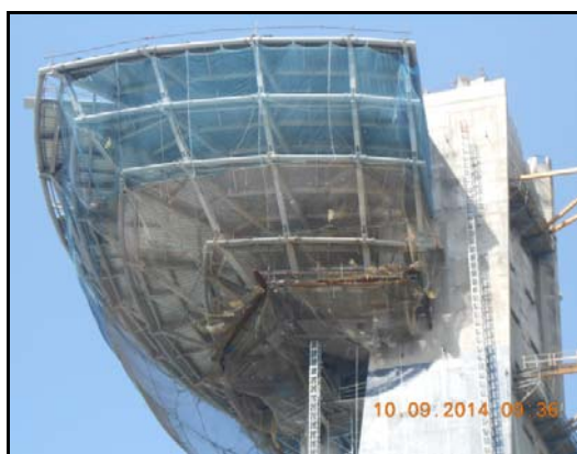
Fig. 1: Field Photo: The observation deck
